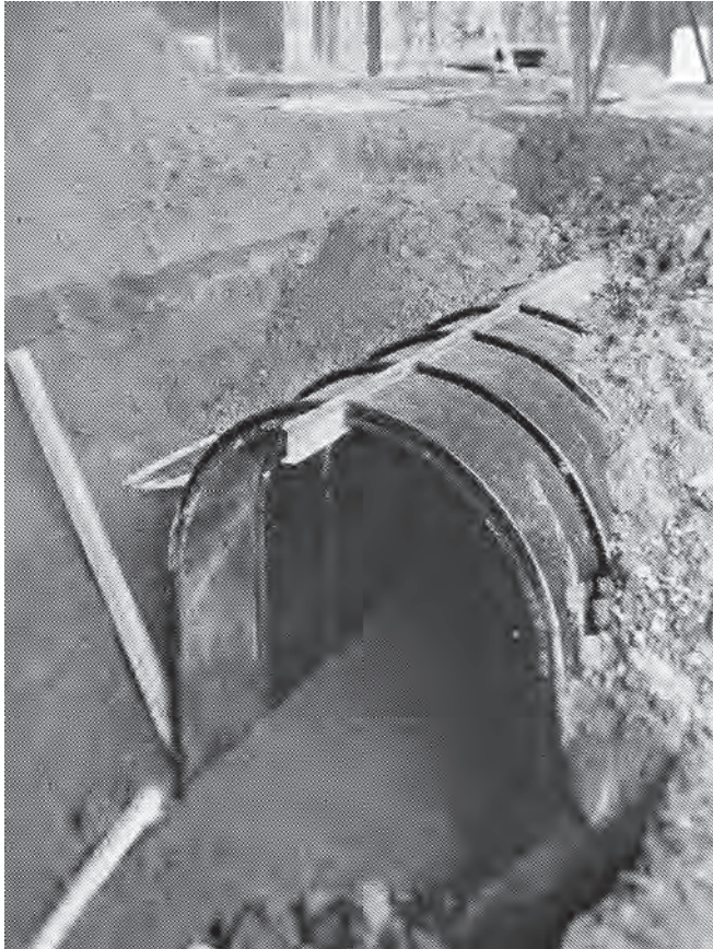
Photo from the brochure of a curved steel sheet shelter similar to the one at Sutton Coldfield.
